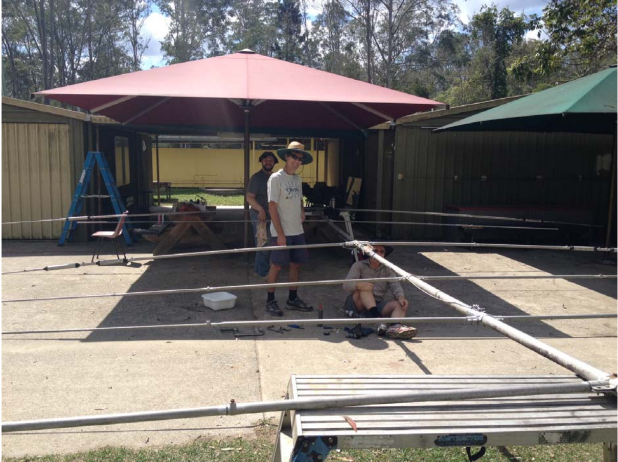
BP Park antenna work
